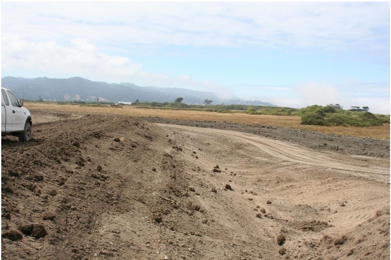
THE SETBACK BERM IS BEING BUILT IN SEVERAL LIFTS
