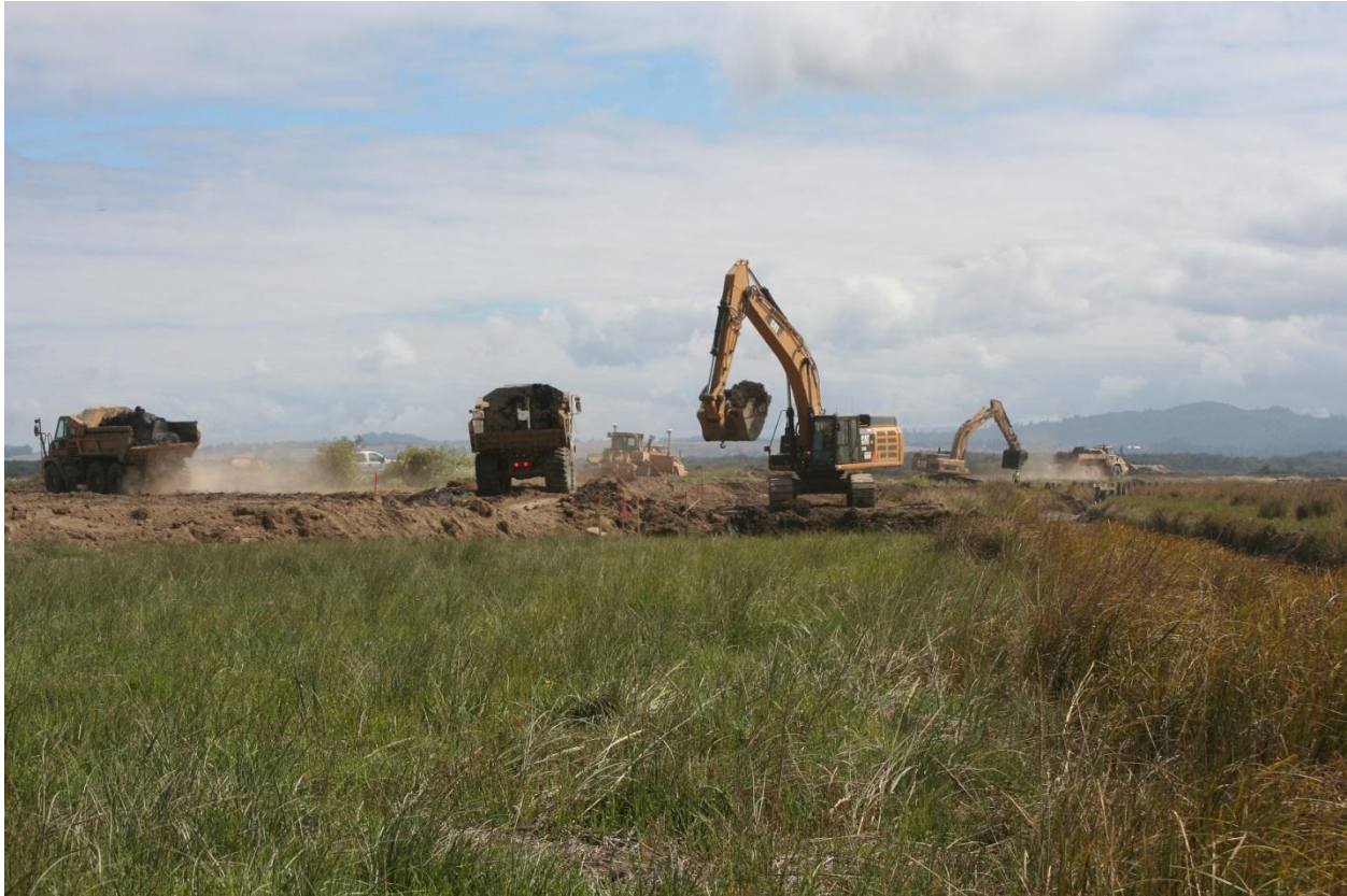
THE SETBACK BERM IS BEING BUILT IN SEVERAL LIFTS
